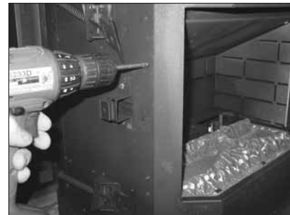
Figure 8.3 To remove existing metal refractory remove the two screws located on the left and the two on the right sides behind the side curtains.
